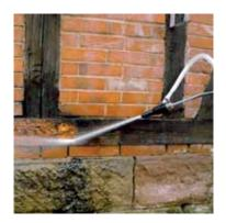
The wet blasting attachment fits easily on Kärcher high-pressure cleaner spray lances. The abrasive is sucked up into the water jet and applied with a powerful abrasive action. Ideal for removing rust, scale and paint from components as well as graffiti.
