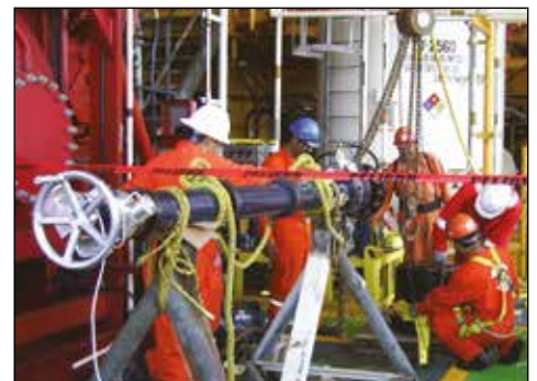
▼ CHT2000 hot tapping offshore application.
